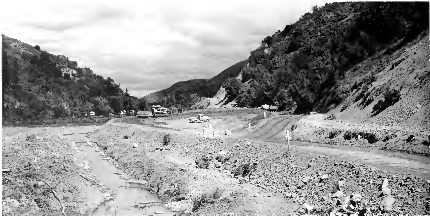
Looking westerly at construction activities on Laurel Dell-Tule Lake project in Lake County at intersection with Scotts Valley Road and at easterly end of Laurel Dell Lake.
